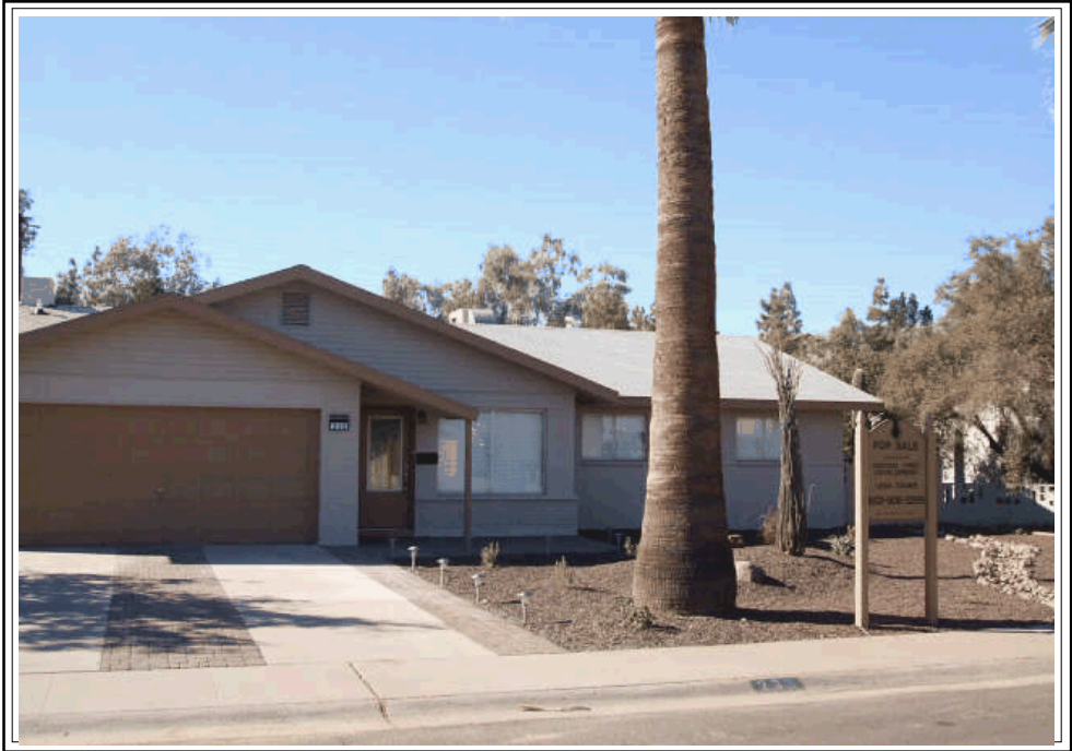
FRONT VIEW OF SUBJECT PROPERTY
